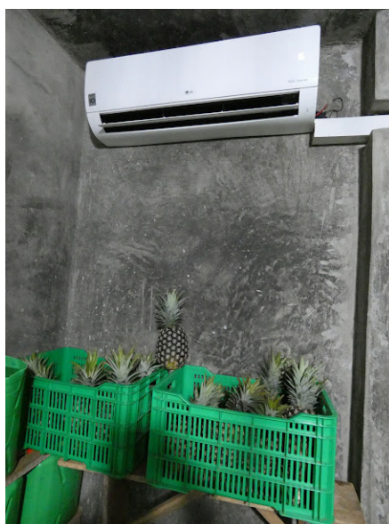
Figure 4: 10*15*6m space cold storage facility. Cooling capacity 2-16 degrees Celsius
